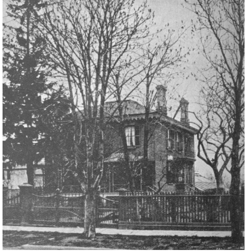
“DON VILLA,” RESIDENCE OF MR. S. H. DEFRIES, BROADVIEW AVENUE.
