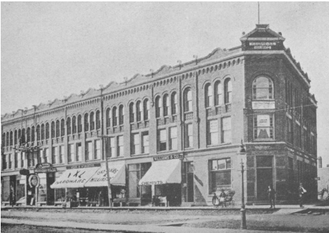
CAMPBELL'S BLOCK, WEST TORONTO JUNCTION.
