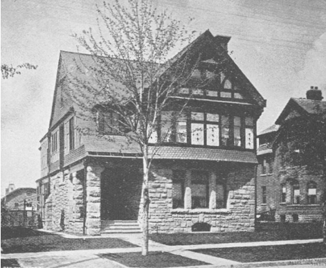
RESIDENCE OF MR. W. E. MASSEY, JARVIS STREET.
