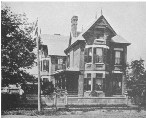
RESIDENCE OF MR. JOHN MALONEY, BROCK AVENUE.
