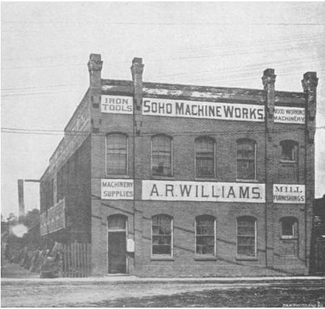
SOHO MACHINE WORKS OF MR. A. R. WILLIAMS.
