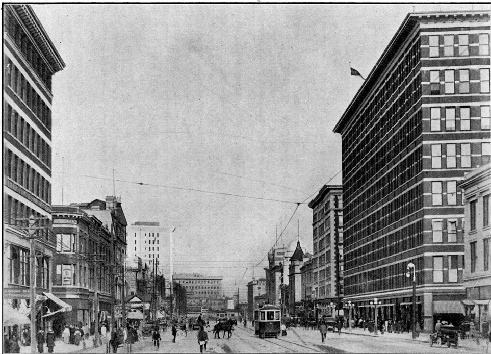
PORTAGE AVENUE, WINNIPEG. LOOKING EAST
