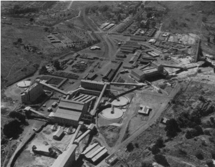
The headgear and surface workings.
