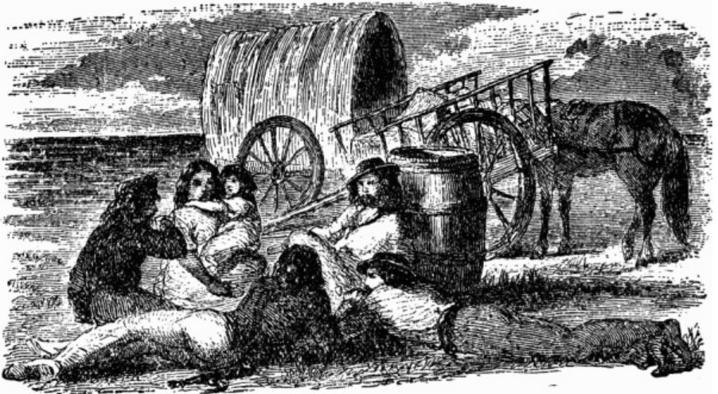
Journeyers across the plains halted for the night.
