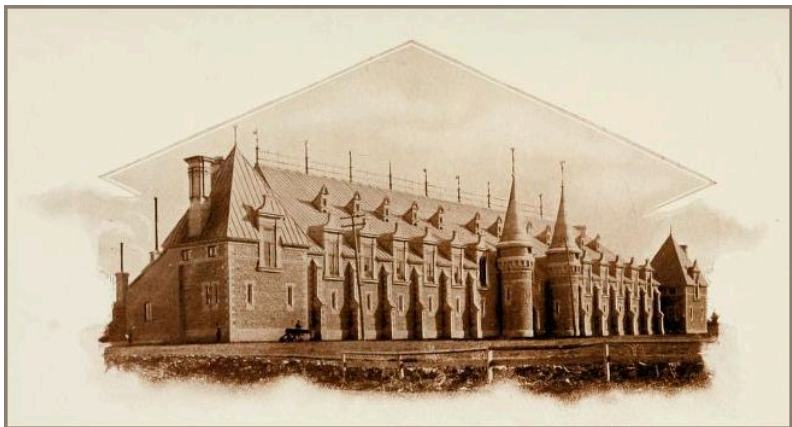
The Drill Hall
