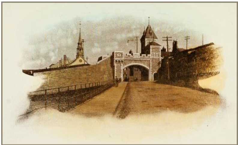
Kent Gate, from the outside
