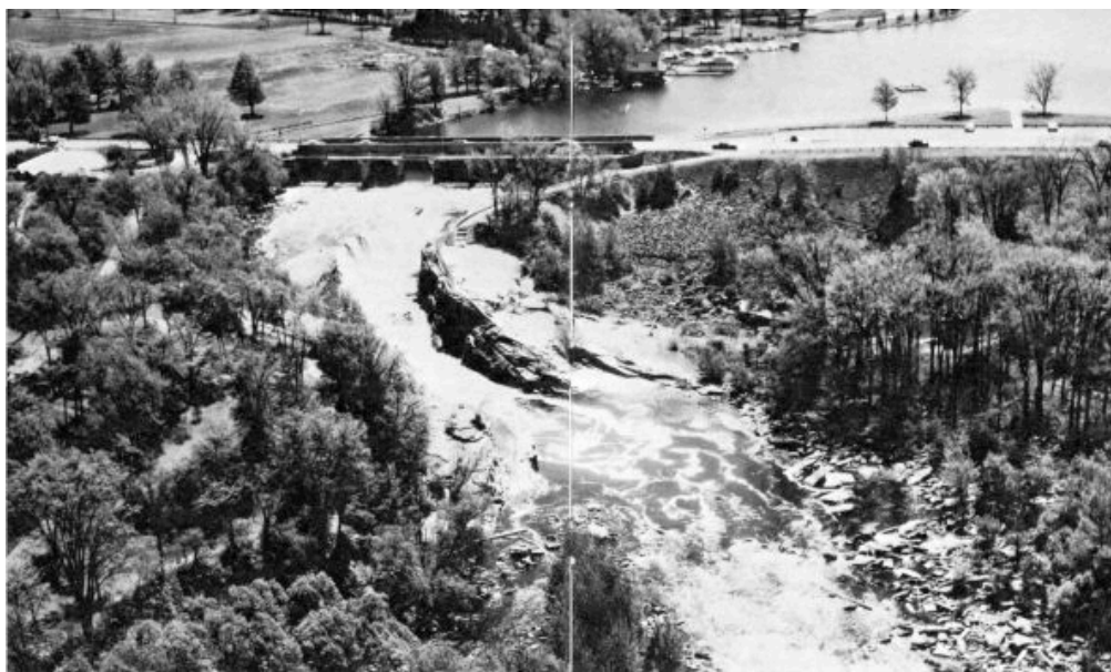
The dam and overflow at Hog's Back. The natural course of the river before installation of the canal system was to the right in the valley bottom.
