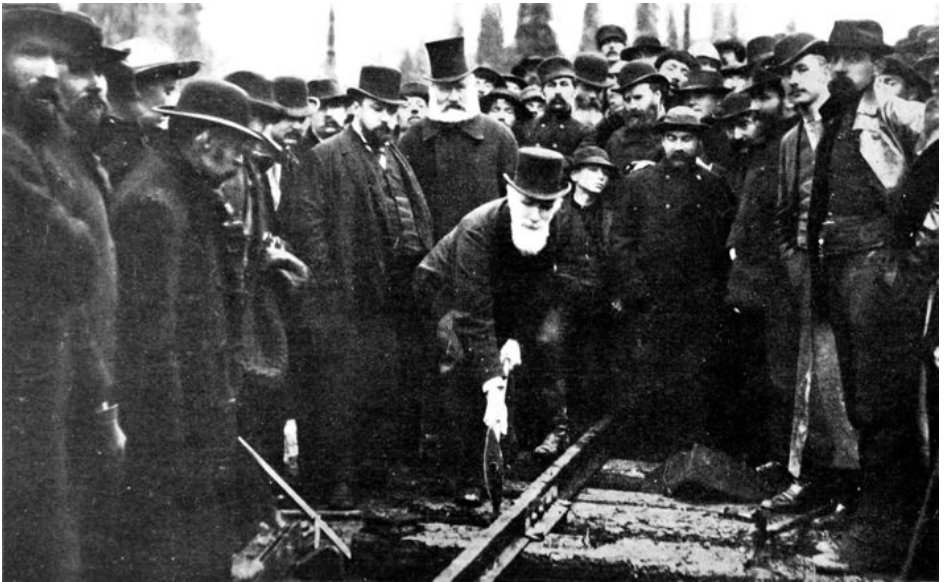
DRIVING THE LAST SPIKE
