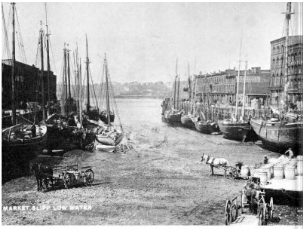
Market Slip, Saint John, at low tide. Right foreground: barrels of lime from a quarry above Indiantown.
