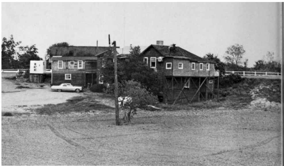
The rear of Giusti's bar and restaurant.
