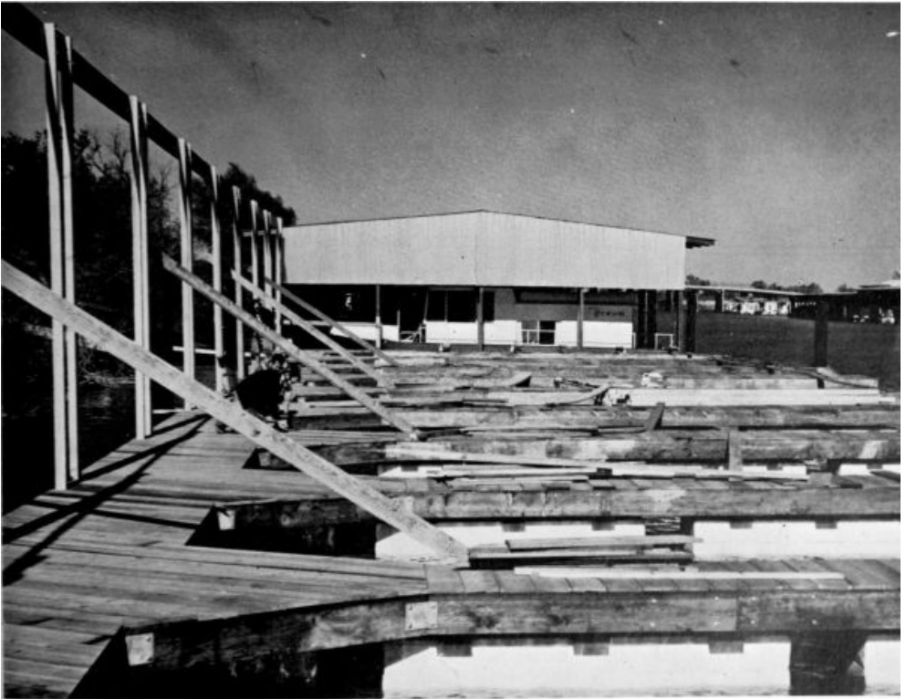
New berths under construction at Remsburg's Harbor.
