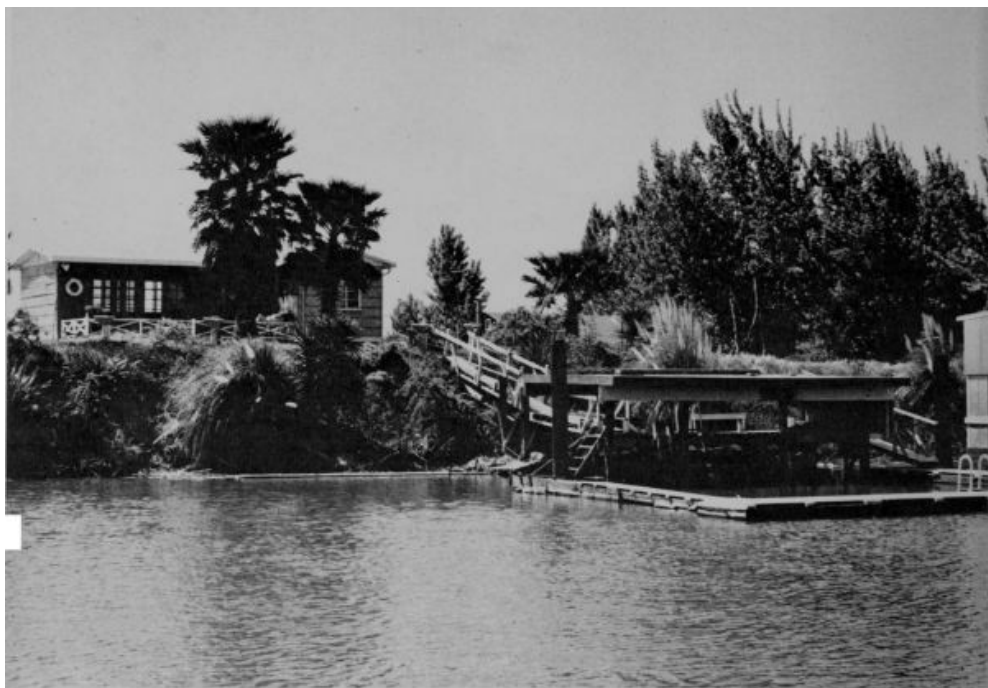
A modern home peers over the levee in Dutch Slough.
