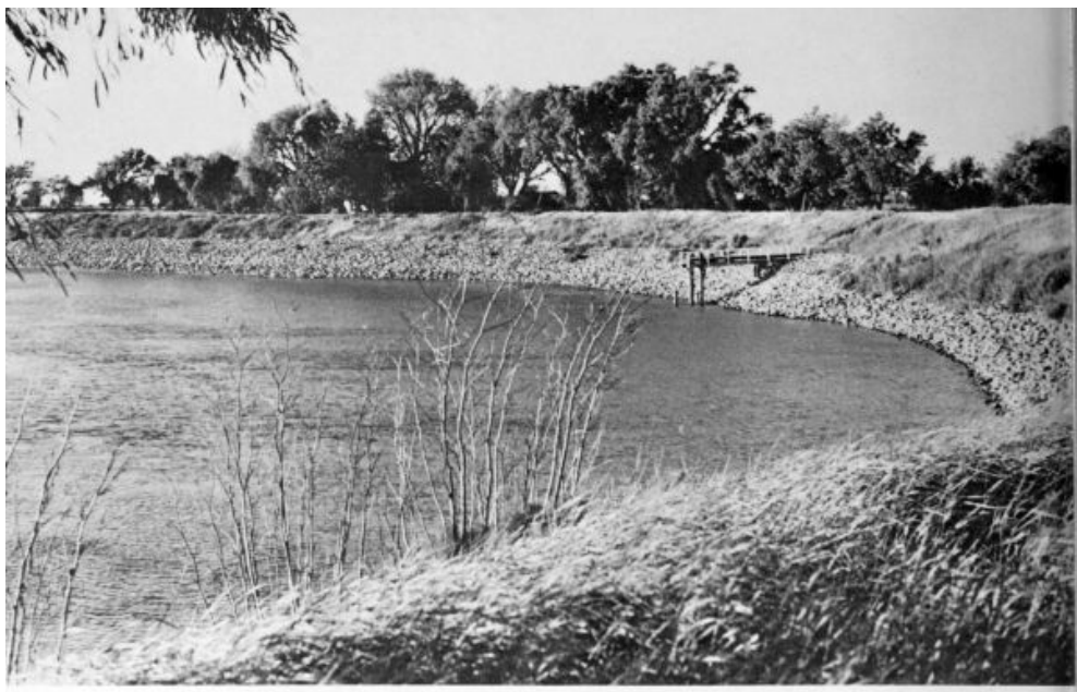
Recently reinforced levee on Steamboat Slough.
