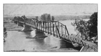
4 Pin Connected Pins 175 Feet Each and 2 Riveted 80 Feet Spans Over Belly River Near Lethbridge.
