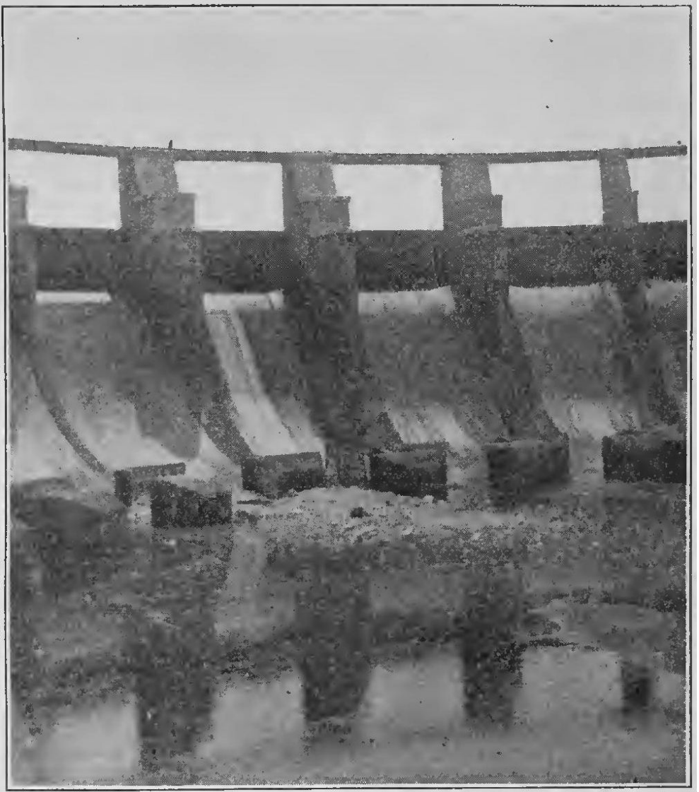
FIG. 4. The spillway of the Gatun Dam
