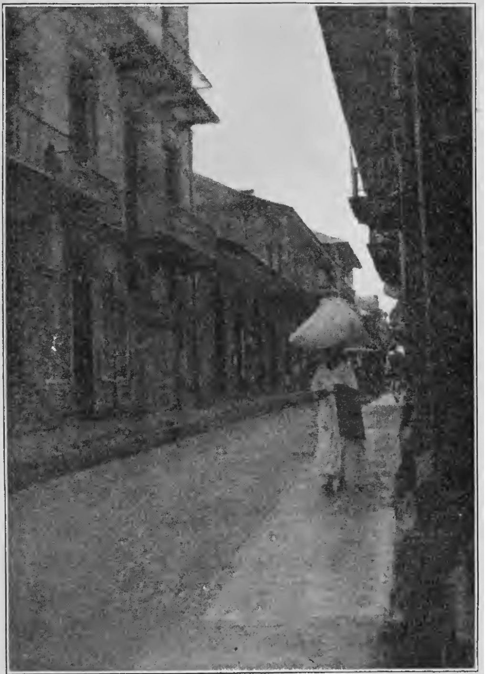
FIG. 80. Clean paved street in Panama
