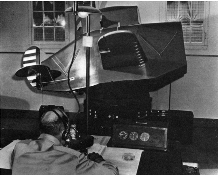
The cadet learns instrument flying inside a Link Trainer
