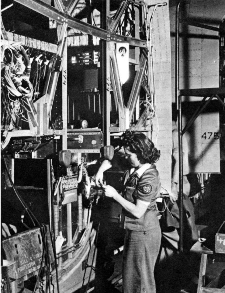
Mid-section of a B-24 on the assembly line
