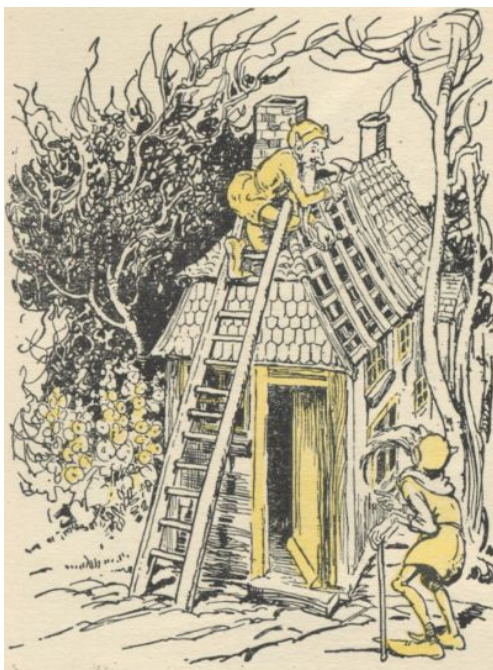
Mickle took a ladder, and spent the whole day mending Winkle's roof.
