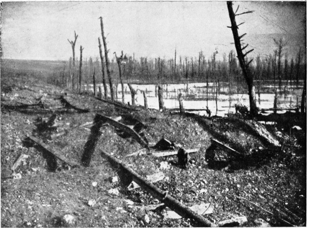
THE RAILWAY LINE AT BEAUCOURT.
