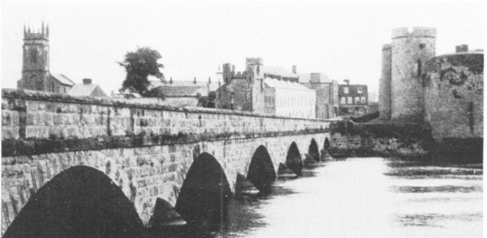
The Thomond Bridge over the Shannon at Limerick City.
