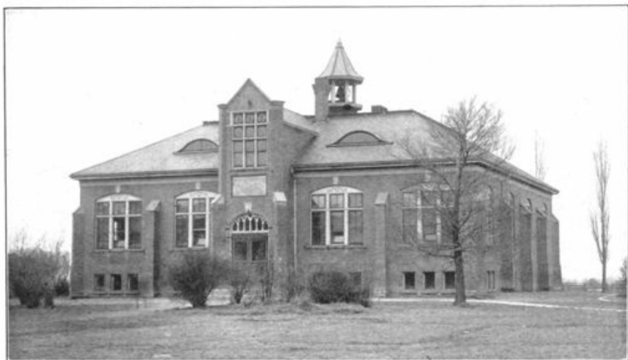
PLAN NO. 14. TWO CLASS ROOMS, WINONA SCHOOL. W. W. La Chance, Architect.
