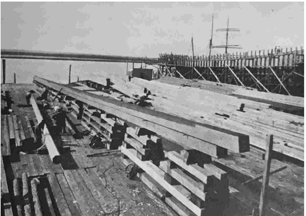
A Wooden Shipyard , showing a Keel on the Blocks.
