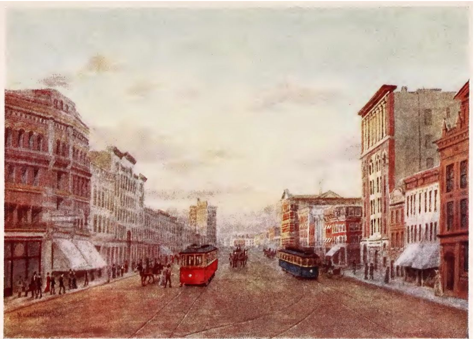
WINNIPEG: CORNER MAIN STREET AND PORTAGE AVENUE
