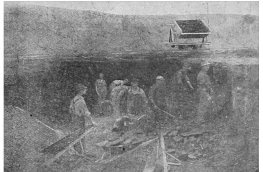
Coal mining at Tofield, Alberta, where an excellent quality is obtained, and where natural gas is abundant.
