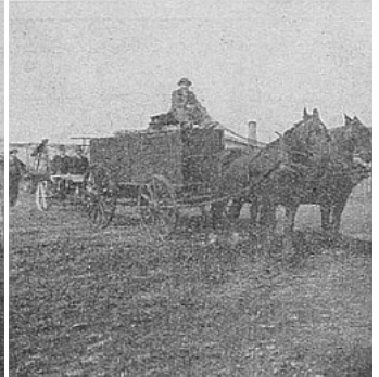
Starting from town with loads of posts for pasture fence.
